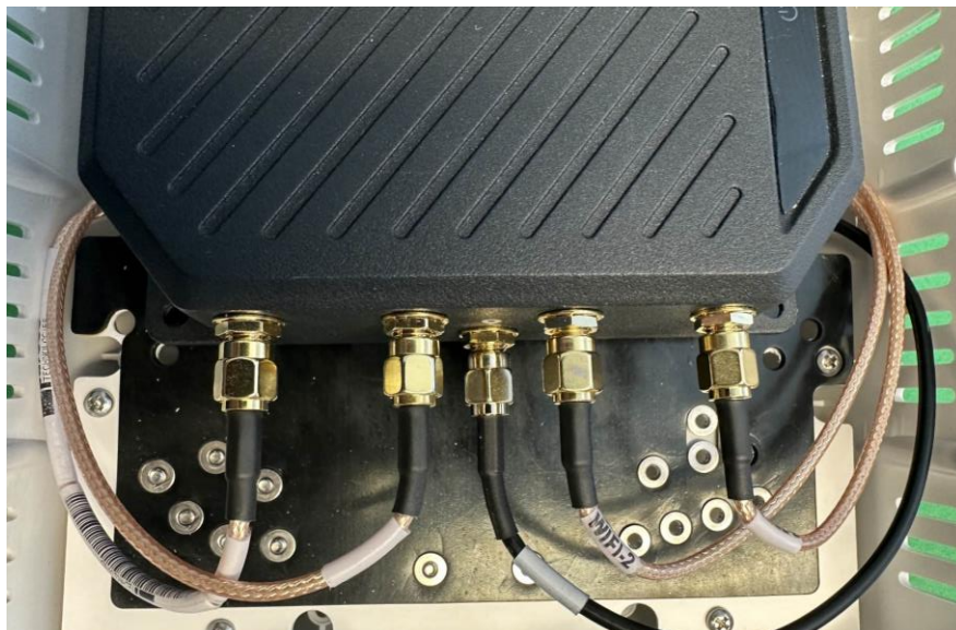
Figure 2: Connecting antenna cables to Router
