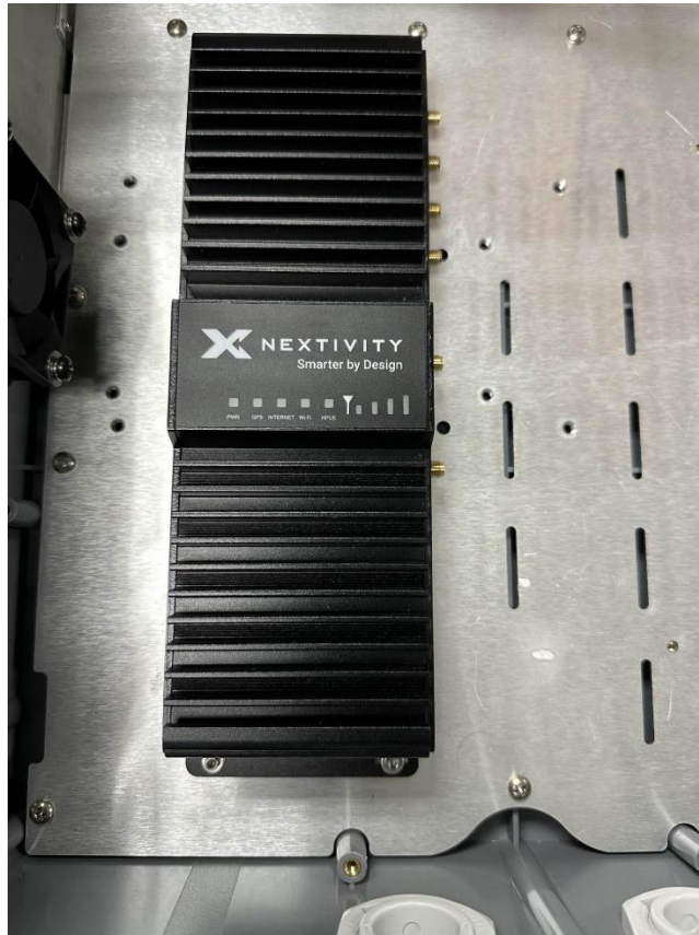
Figure 10: Nextivity SHIELD MegaFi Router Installation
