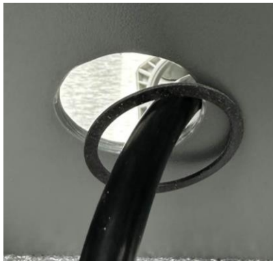
Figure 17: Feeding the gasket through the cable
