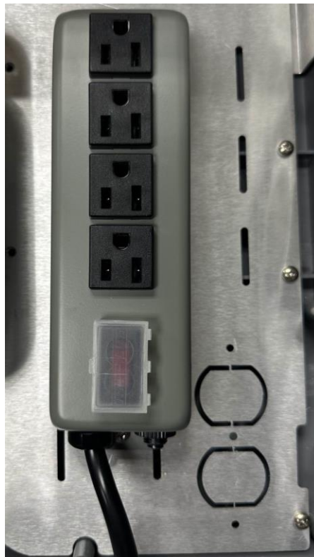
Figures 18-20: Power Strip Installation
