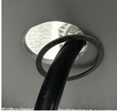
Figure 25: Feeding the gasket through the cable
