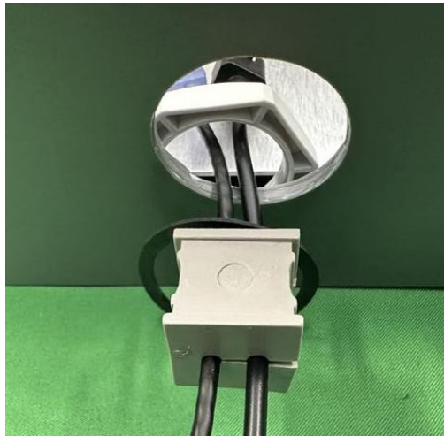
Figure 19: Installing the cables into the grommet
